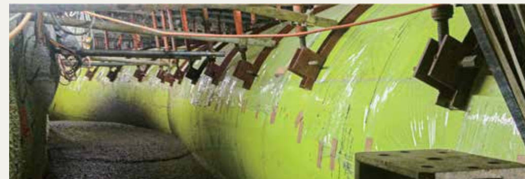
Project Owner: Drainage Serices Department Of HKSAR Details: Provision Of FRP Formworks To The Concreting Of Sewage Conveyance System From North Point To Stonecutters Island. Across Victoria Harbour
